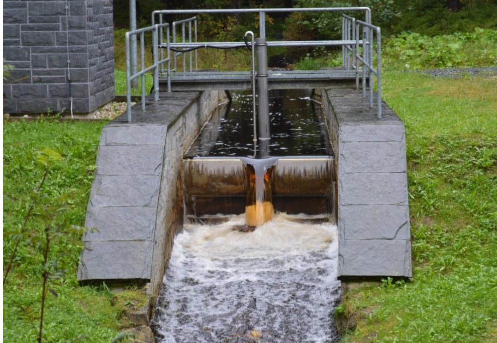
Photo: A stream with heavily coloured brown water after a rain event. Muldenberg, September 2014. Photo by Tallent Dadi
