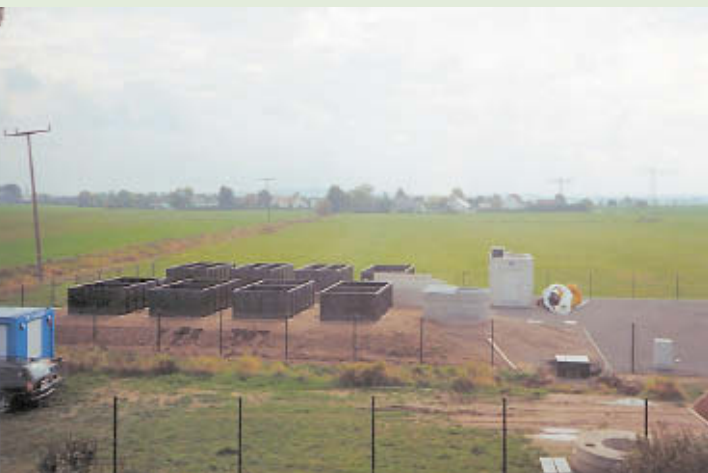
Langenreichenbach pilot plant during construction – 1
