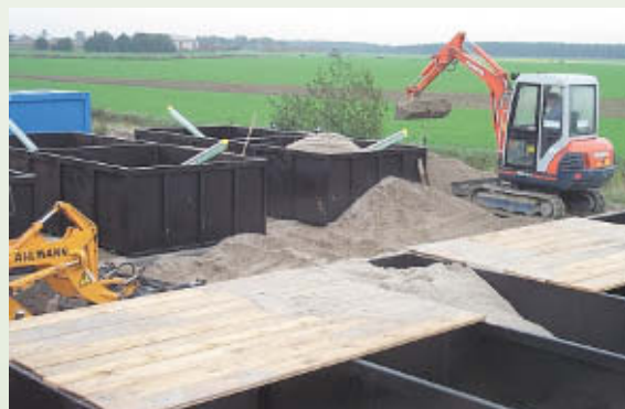
Langenreichenbach pilot plant during construction – 2
