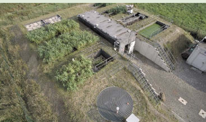
Pilot plant “Langenreichenbach”, Germany
