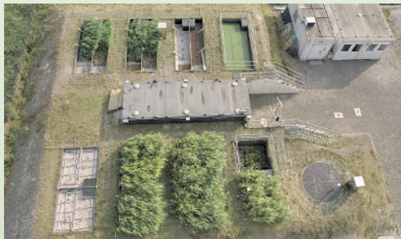
Top view of the completed experimental plant
