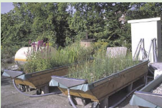
Mobile test unit of horizontal flow filter
