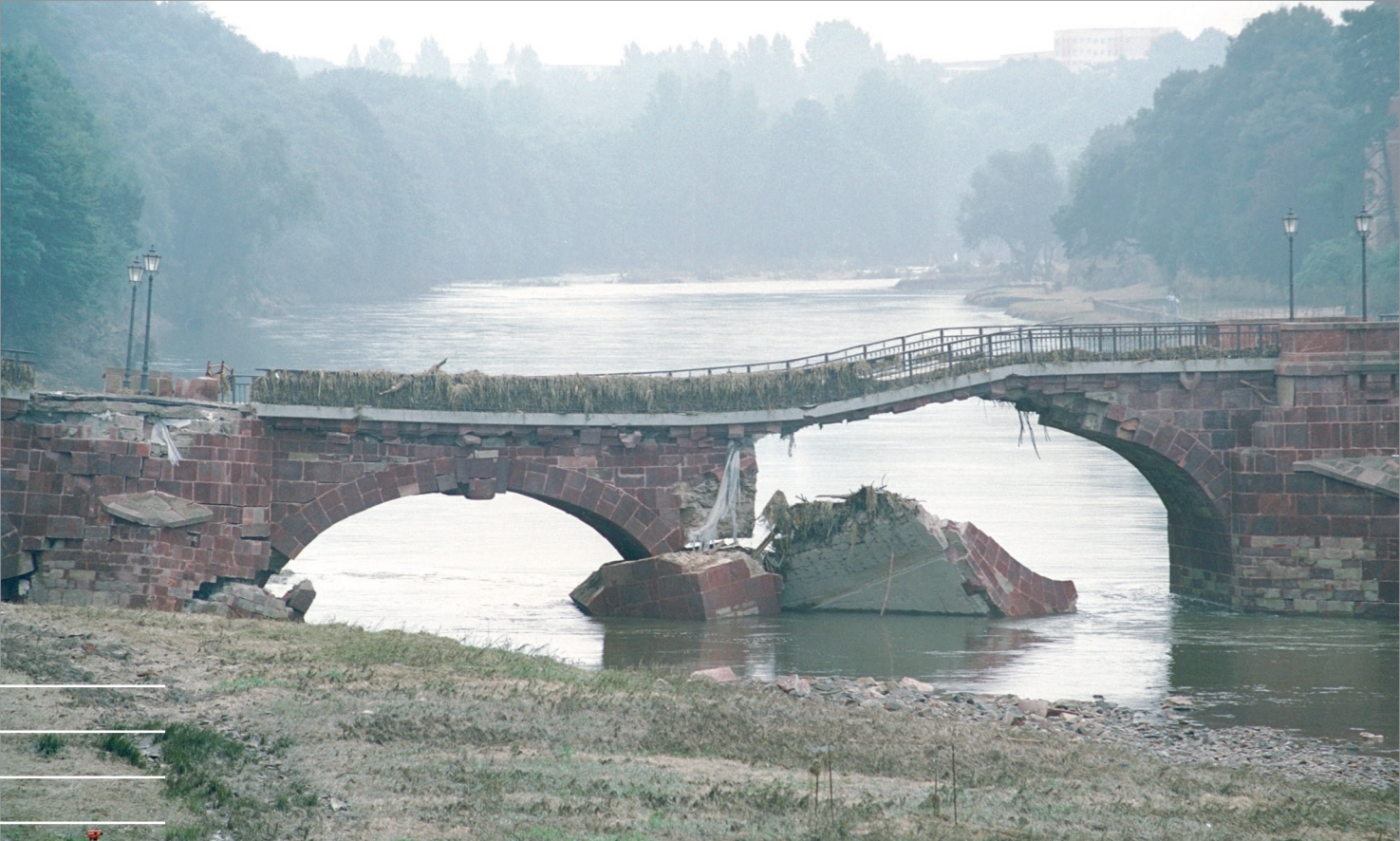
05 Destroyed Pöppelmann Bridge in Grimma after the 2002 Mulde flood Photographer André Künzelmann
