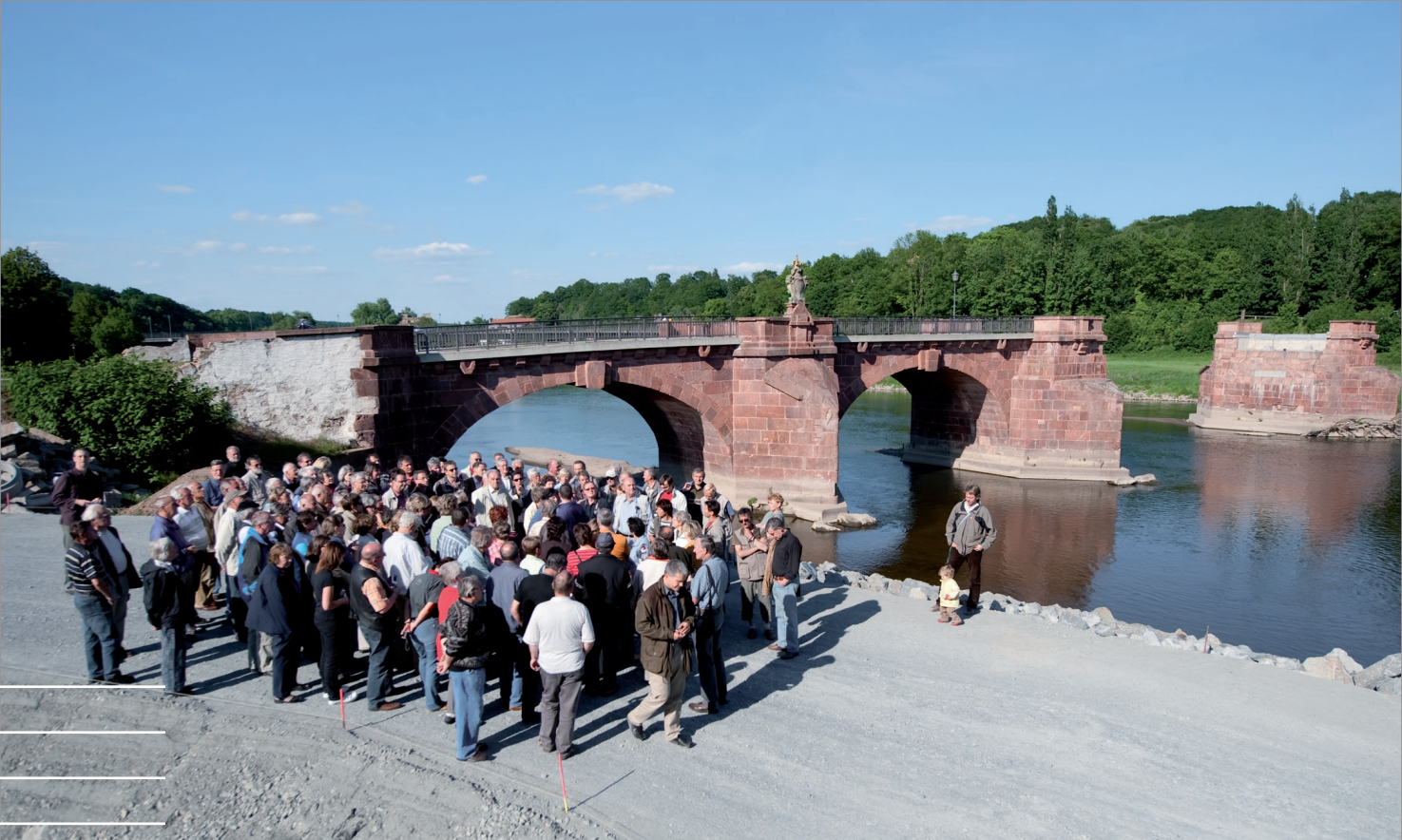
10 Informing the public about the new flood wall in Grimma 2009 Photographer André Künzelmann
